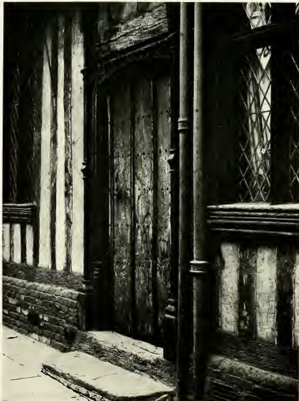
OLD OAK HOUSE, SIDE ENTRANCE DOOR
